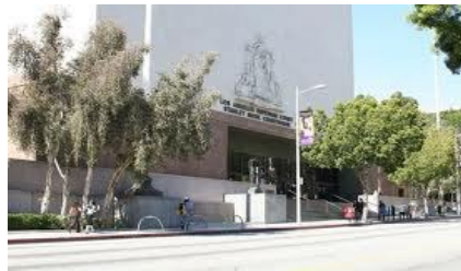
Stanley Mosk Courthouse in Downtown Los Angeles
